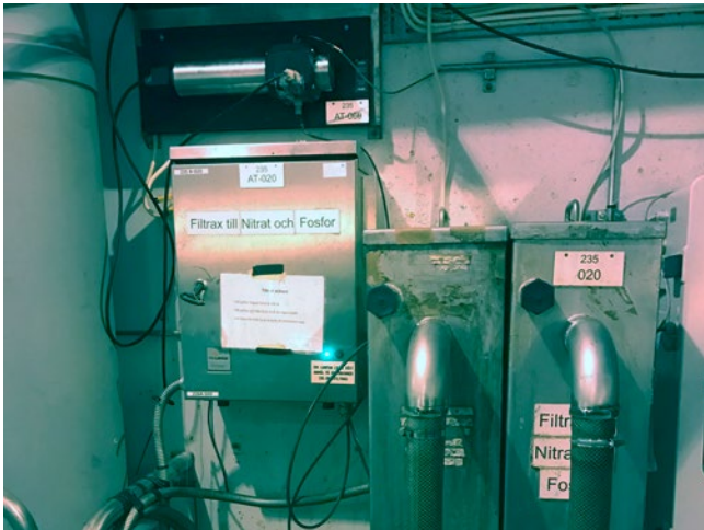
Pictured top left is the Nitrate analyser Nitratax plus mounted in a flow-through fitting and below that you can see the Filtrax unit and the boxes where the filter is mounted.
